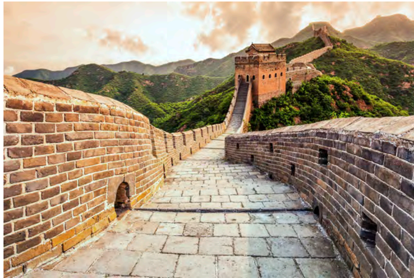
Image 5: Construction of the Great Wall.
